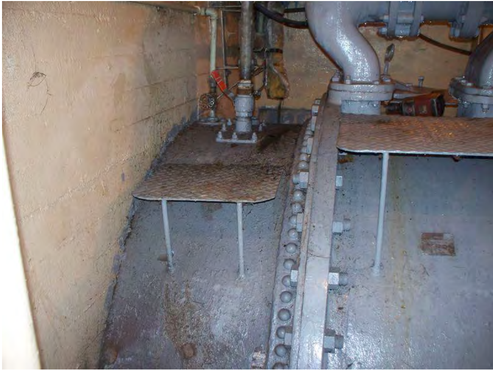
Penstock at concrete wall top side
