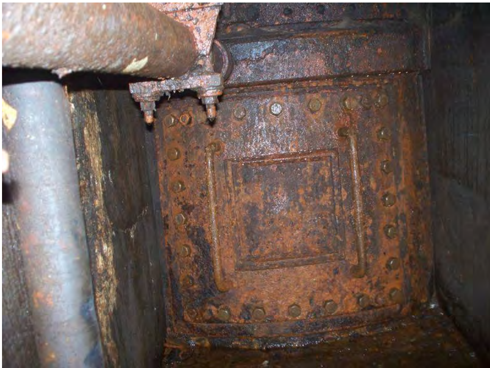
Draft tube access hatch, general surface corrosion noted
