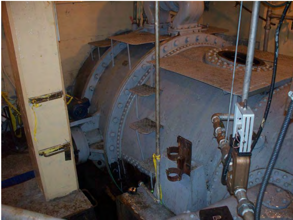
Unit 3 penstock, butterfly valve to scroll
