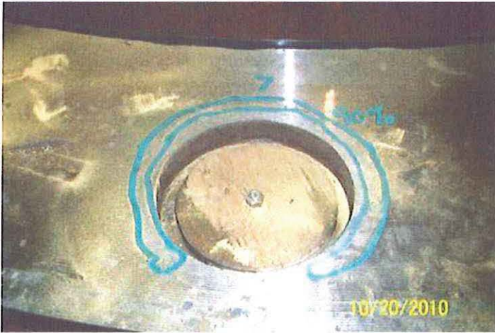
HOLE #7 WITH LINEAR INDICATION 90% AROUND HOLE
