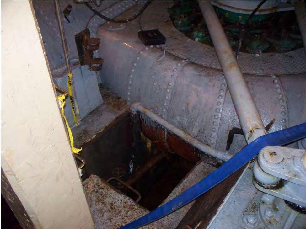
Scroll case – draft tube access area
