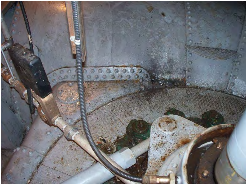
Top side view of scroll – good general condition, minor corrosion/pitting at edge of checker plate on scroll
