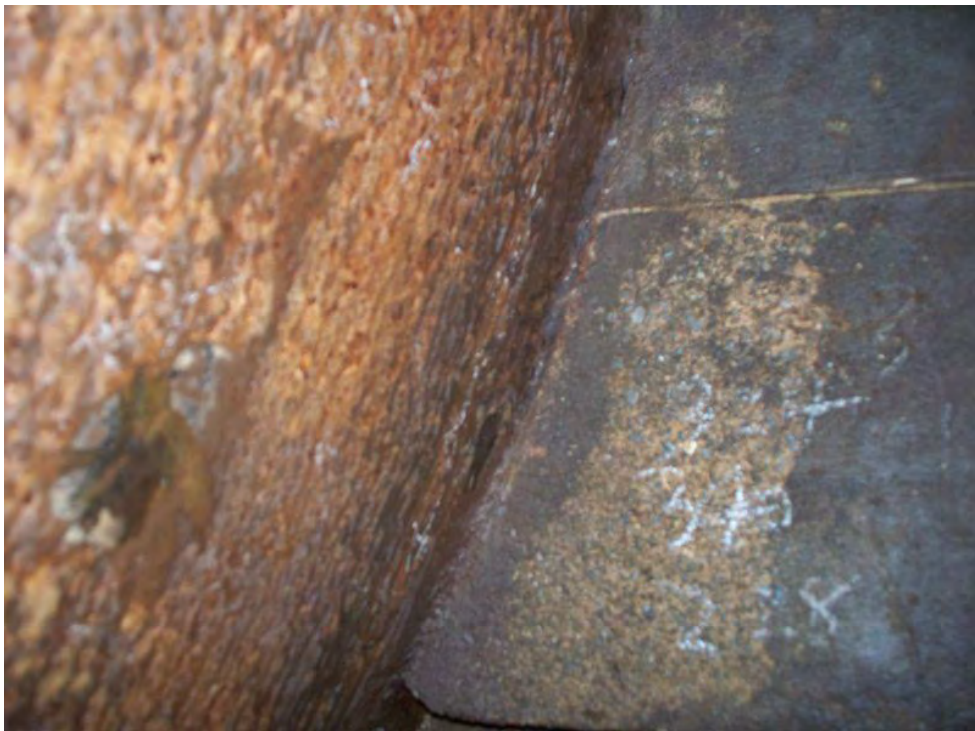
Penstock opposite side at concrete wall – significant corrosion noted
