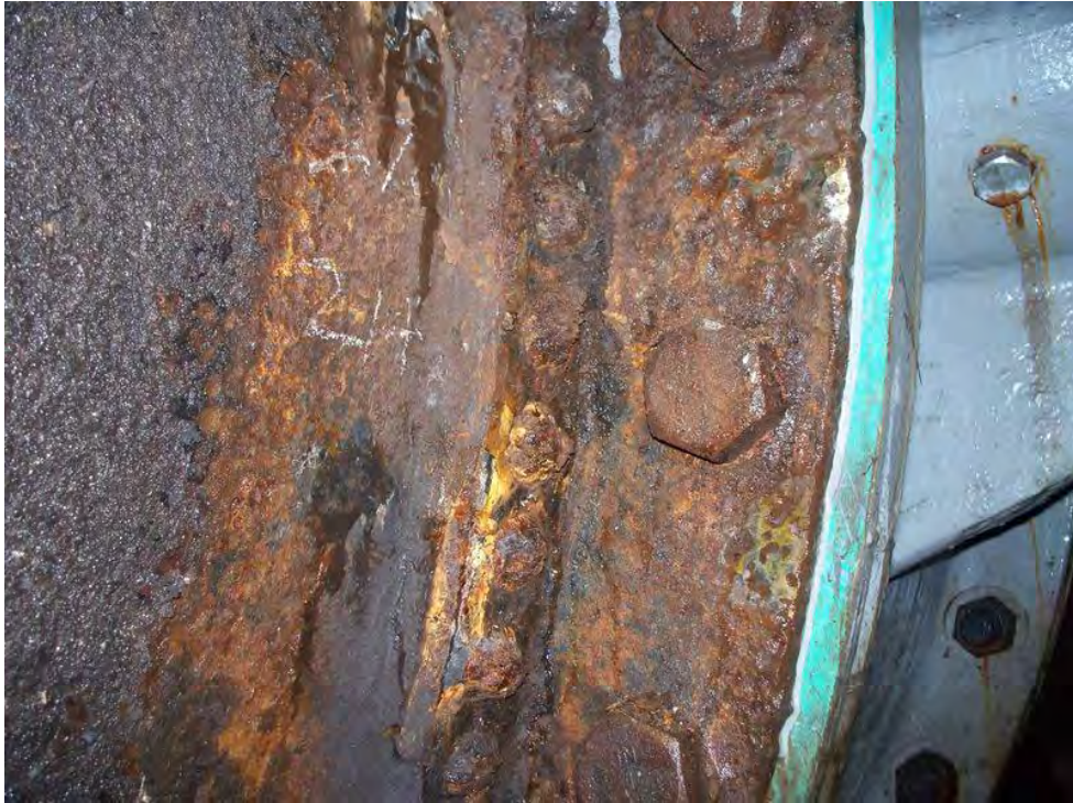
General corrosion just below area viewed in photo 3288. Flange and penstock corroded significantly
