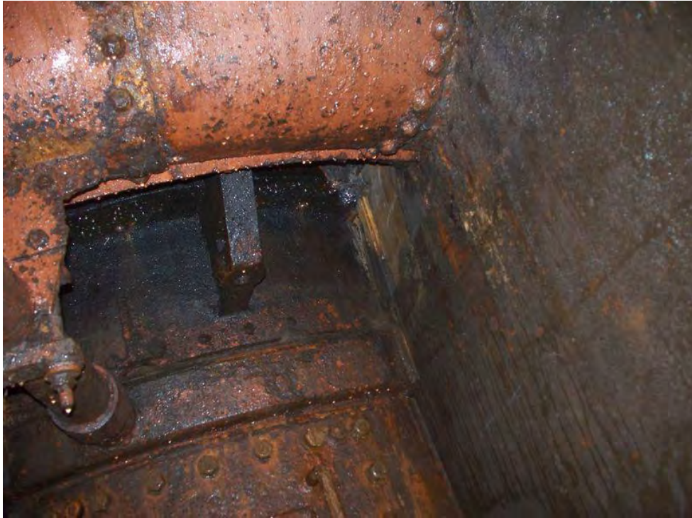
View upward from hatch – note 5 rivets missing at joint above hatch
