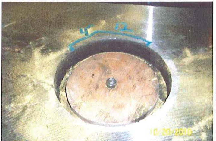
HOLE #12 WITH 4" LINEAR INDICATION AROUND HOLE
