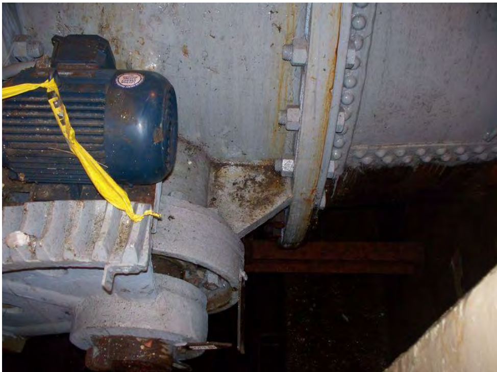
Control side of butterfly valve – cracks noted at gusset/stiffener to upstream and downstream flange, both sides, 4 areas in total
