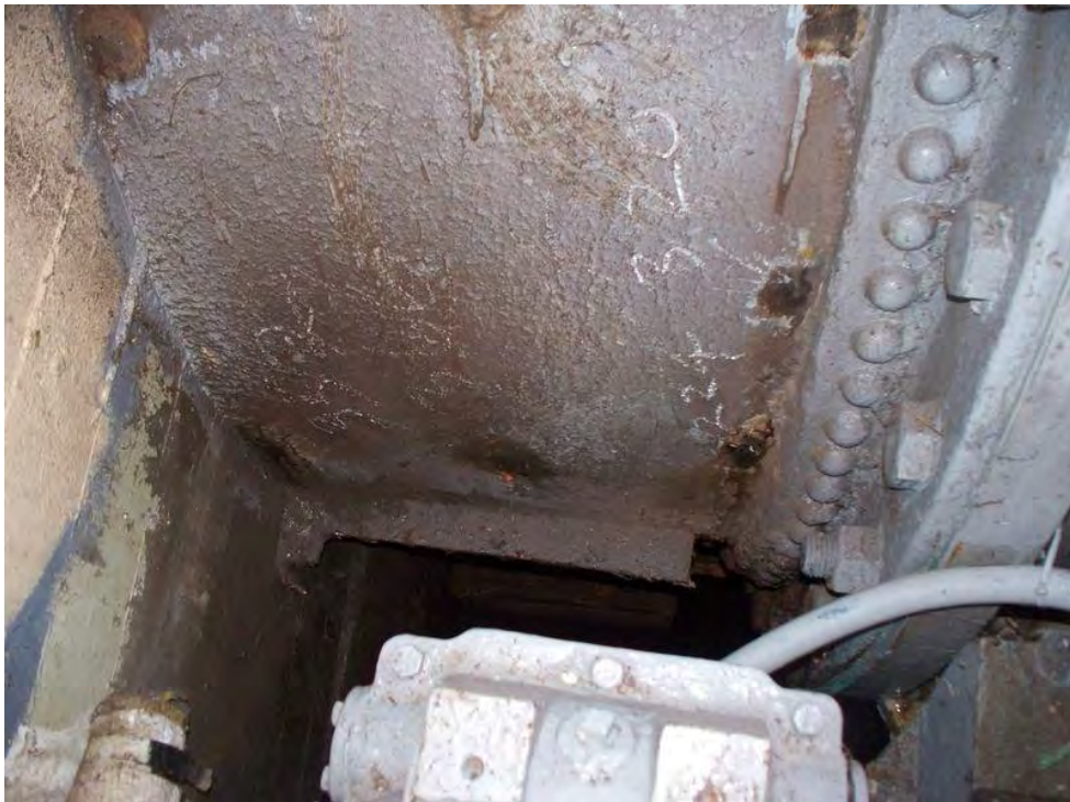
As above, side view, corrosion noted at lower areas per report info
